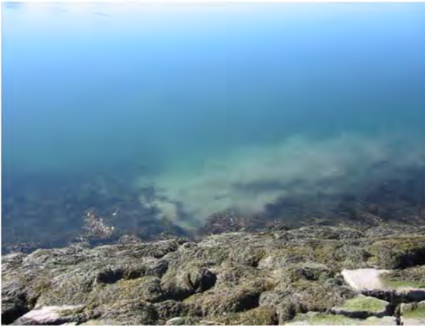
Figure 3: Inadvertent drilling fluid return in waterway
